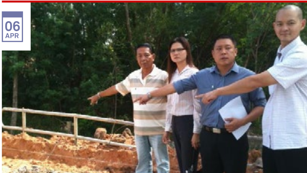
▲ Inspecting a land erosion case in Taman Seri Bahagia, Cheras with Balakong ADUN Eddie Ng.
